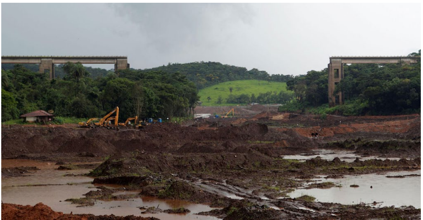
Vale’s tailings dam in Brumadinho
